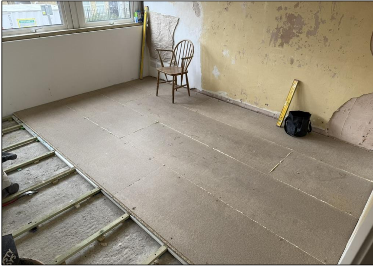
But the new floor needed a multi-skilled renovation by my fast-becoming friend Dan! The timbers here show how he levelled the floor and laid insulation below flooring.
