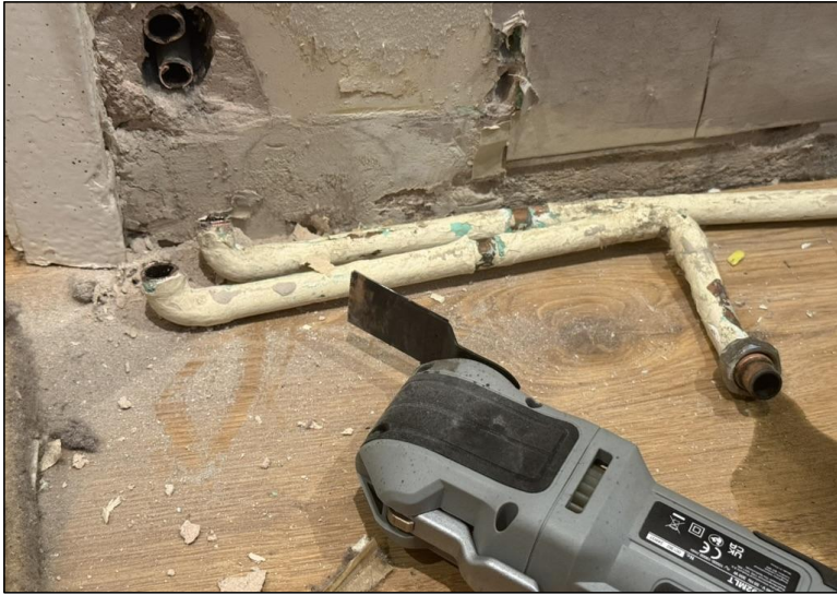
New tool for cutting out old pipes.
