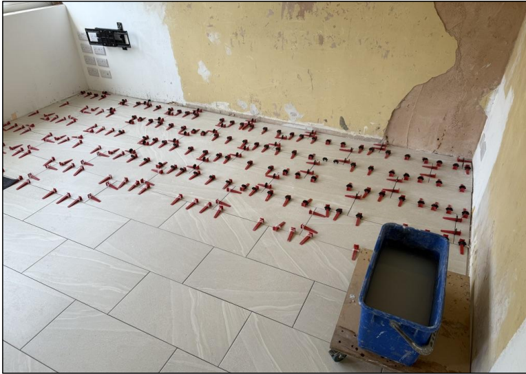
And finally tiling all over.
